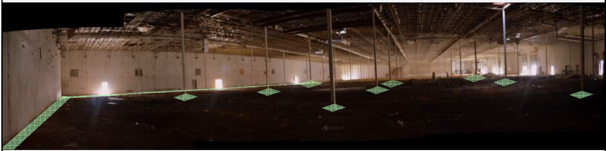
Chemically Injected Areas (15' Below Grade)
