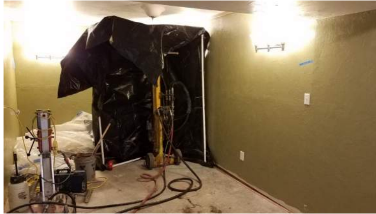
Interior Installation of Grout Pipe with Very Small Drill
